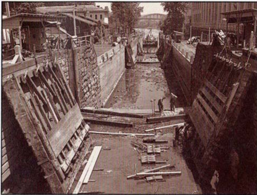
As part of the 1940s restoration, the original wooden lock gates were replaced with metal gates.
