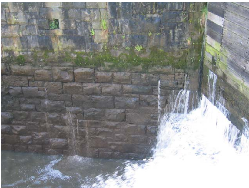
Photo 3-3 Through Wall Leakage (Riverside) (Flow path continues to lengthen as the chamber fills)
