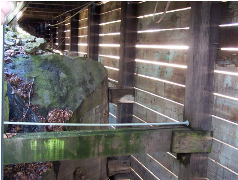
Photo 3-12 River Side - Chamber 1 Wall Anchors and Timber Framing
