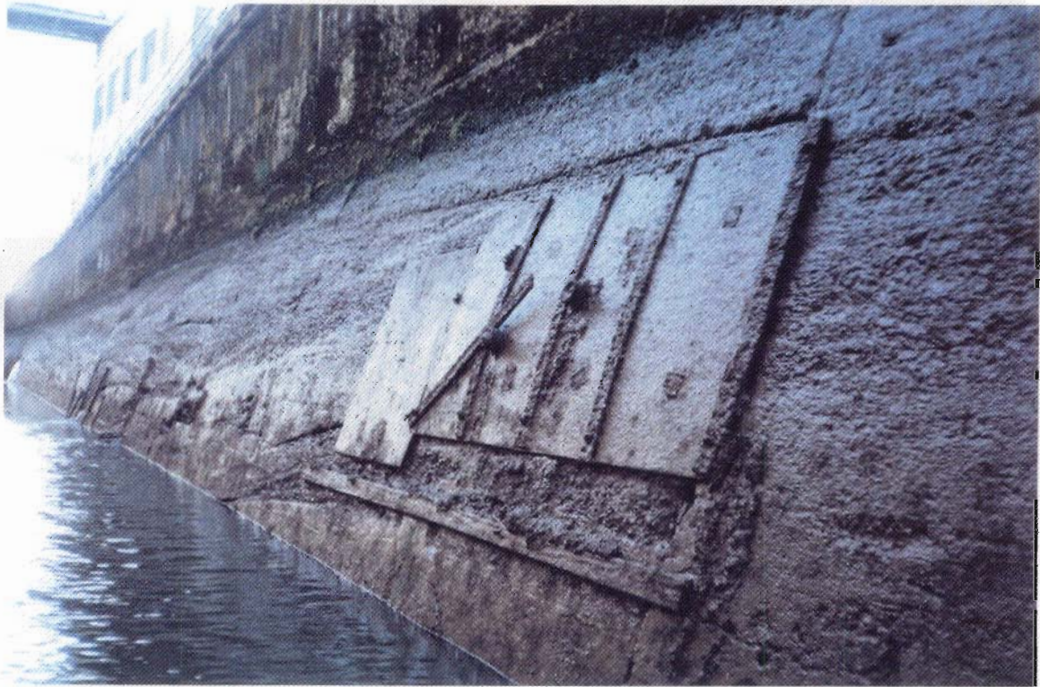
32. Concrete wall on right side of canal at PGE forebay, note former repair areas.
