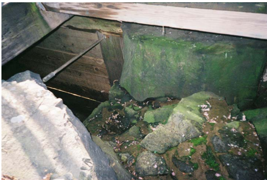
Photo 3-13 River Side - Chamber 1 Wall Anchor
