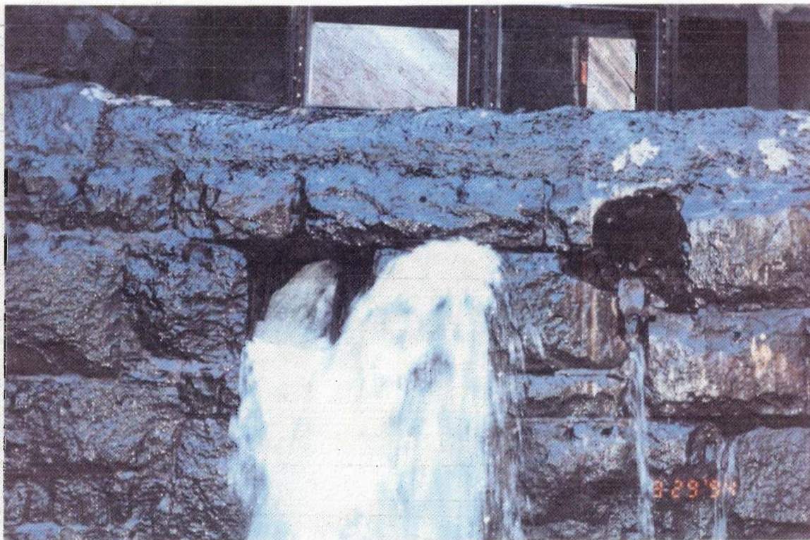
12. Gate 3 sill, right side, missing blocks (bypassing sump)
