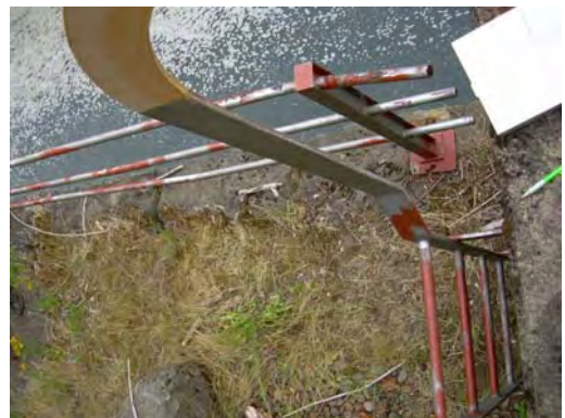
Various Handrail deficiencies at the Willamette Falls Locks
