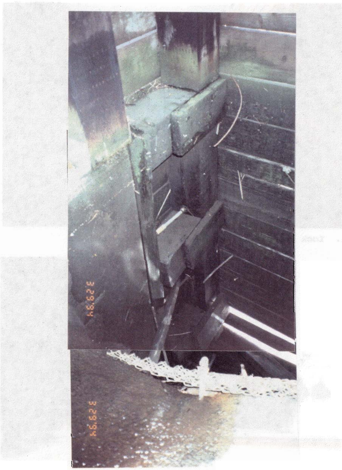
3. Split timber in lock 1, corner post upstream of gate 1, left side.
