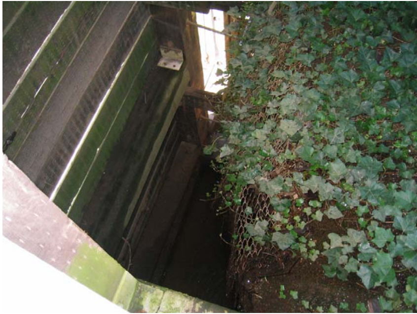
Photo 3-11 Land Side - Chamber 1 Face of Rock Cut, Wire Fabric on Upper Portion and Timber Lining
