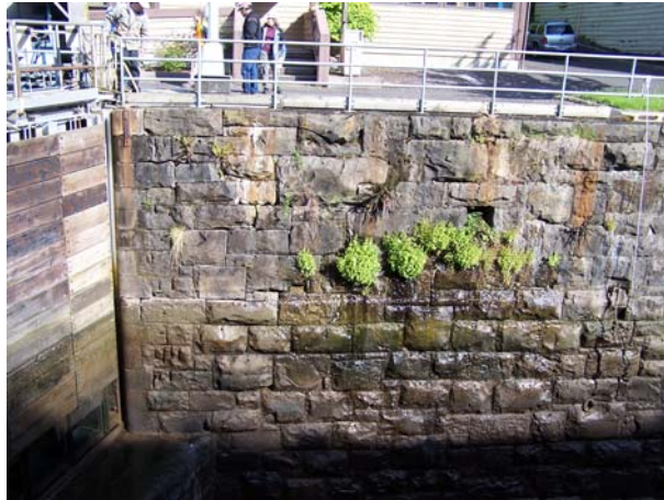
Photo 3-4 Through Wall Leakage (Landside) / Prior to Filling Upstream Chamber
