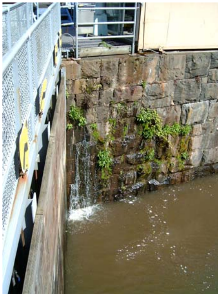
Photo 3-5 Through Wall Leakage (Land Side) (Enough soil has been washed into the joints to support vegetation)
