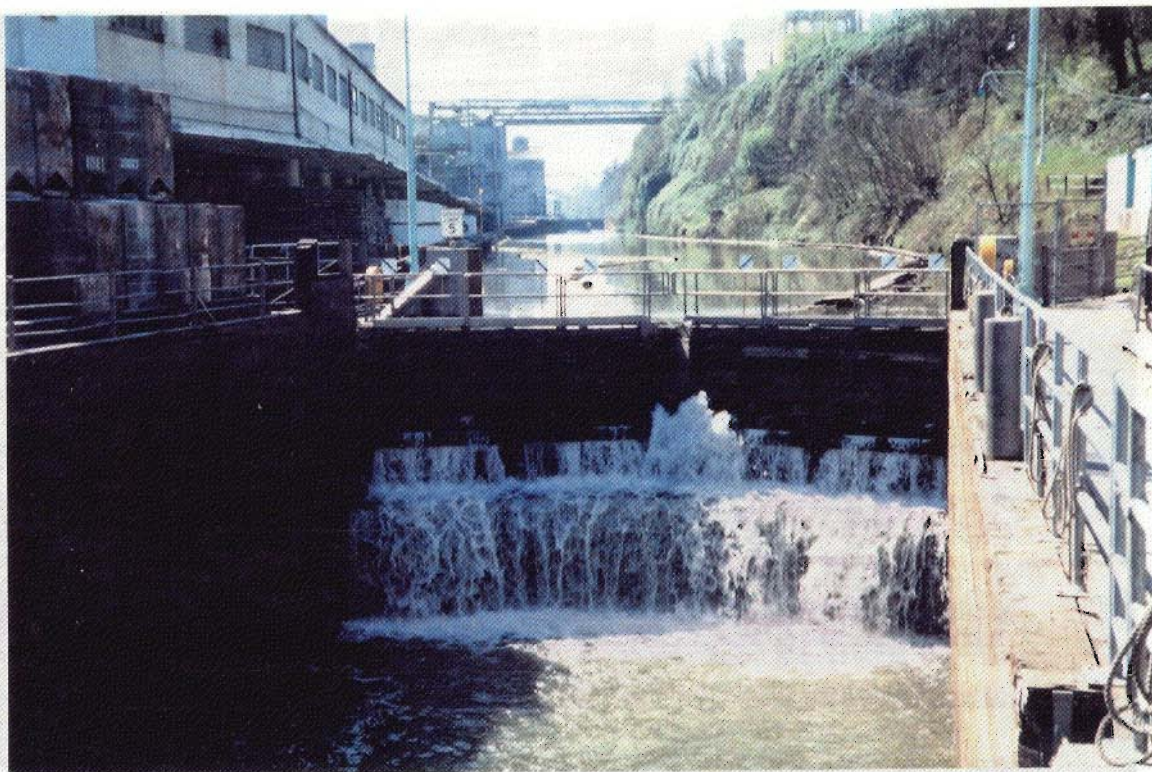
26. Gate 5, downstream face after closing, water level rising upstream of gate.
