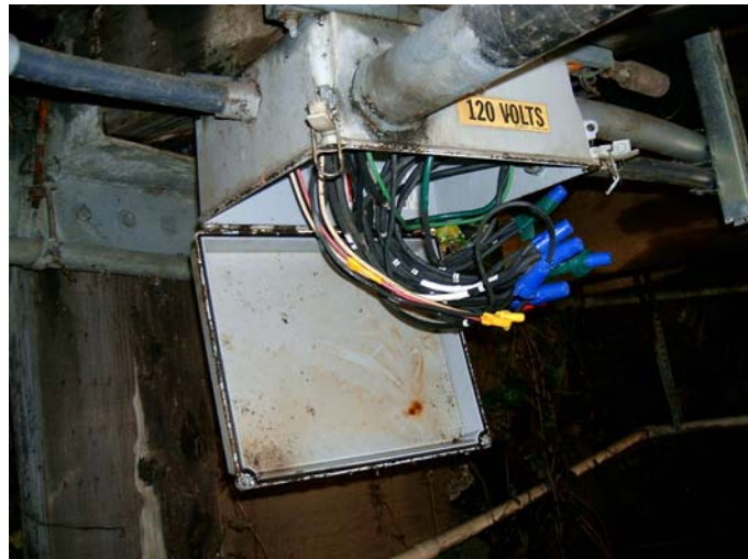
Photo 4-2 Junction Box Contained Water When Opened
