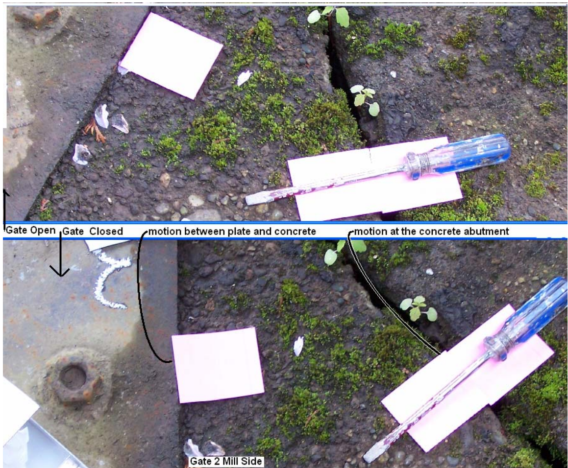
Photo 3-25 Motion Observed between Open and Closed Position, Gate 2
