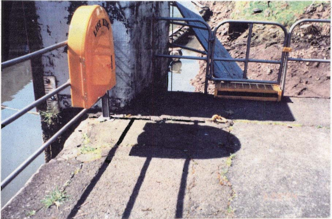
28. Upstream of gate 5, loose concrete guide block (1/2-inch separation between block and asphalt).
