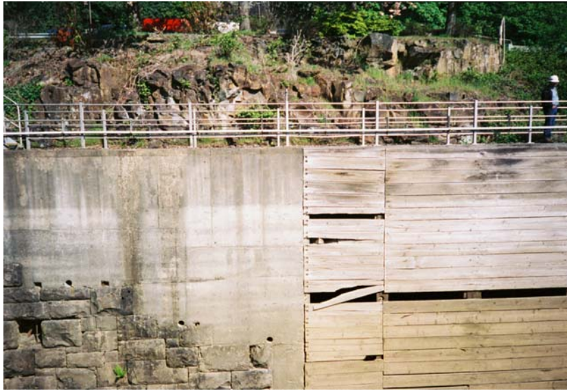
Photo 3-22 Landside Wall - Downstream Approach (Note missing wall facing and core holes for wall anchors)
