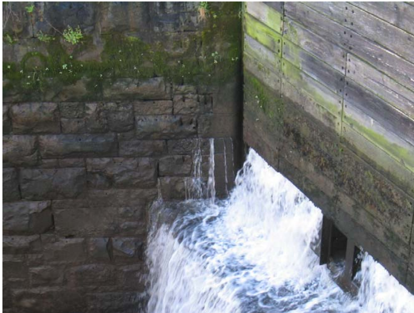
Photo 3-1 Through Wall Leakage (Riverside) (Flow initiates as the chamber begins to fill)
