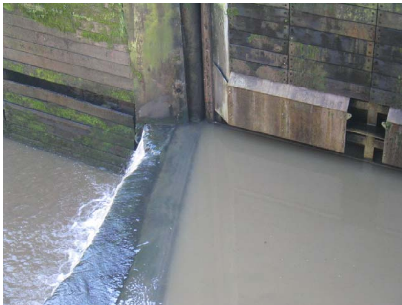
Photo 3-23 River Side Wall - Chamber 1 One Board Missing
