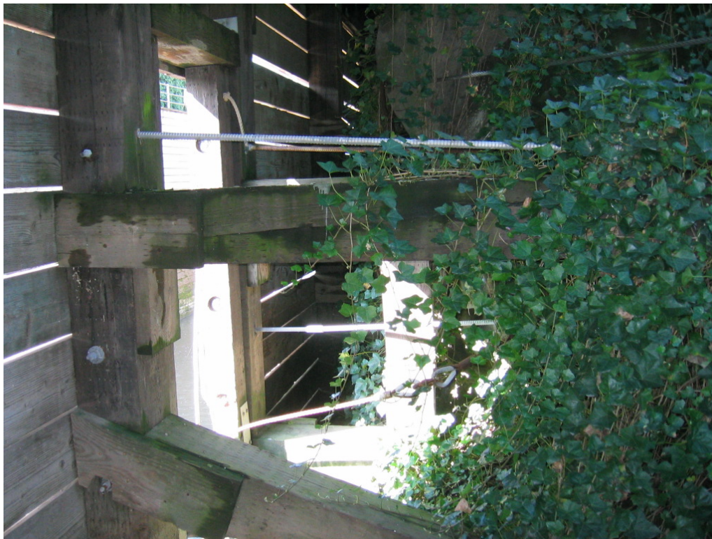
Photo 3-10 Land Side - Chamber 1 Wall Anchors and Timber Framing
