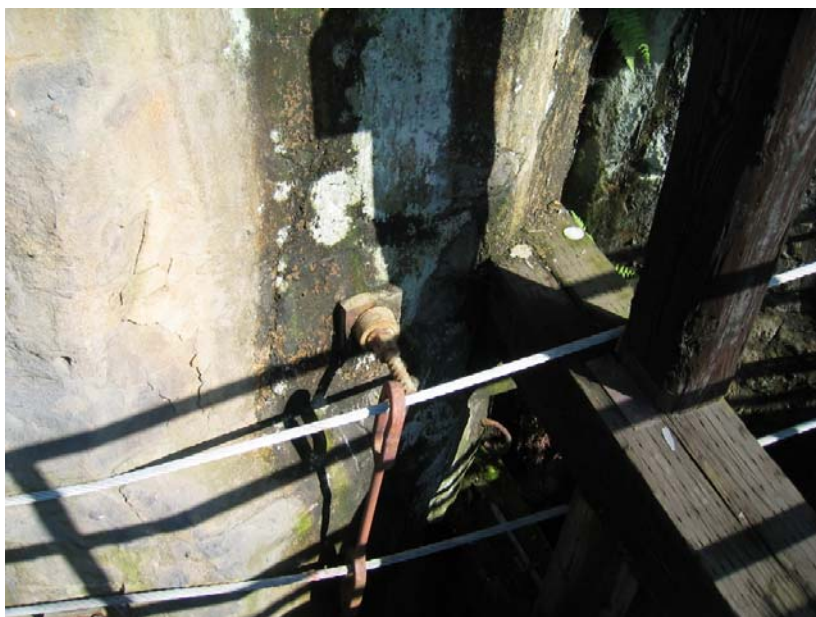
Photo 3-14 Land Side - Chamber 1 Rock Bolt
