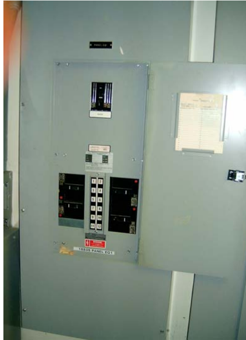
Photo 4-1 480V Panel Board Providing Power to Locks
