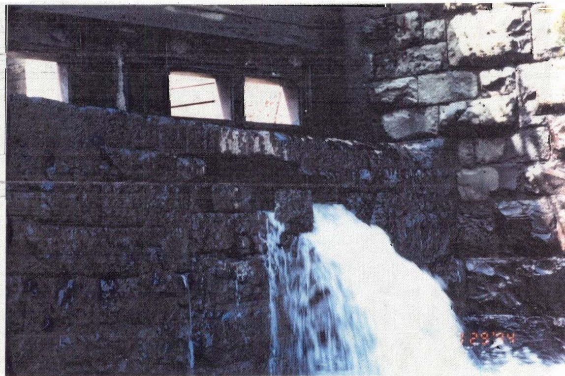
13. Gate 3 sill, left side, missing blocks.
