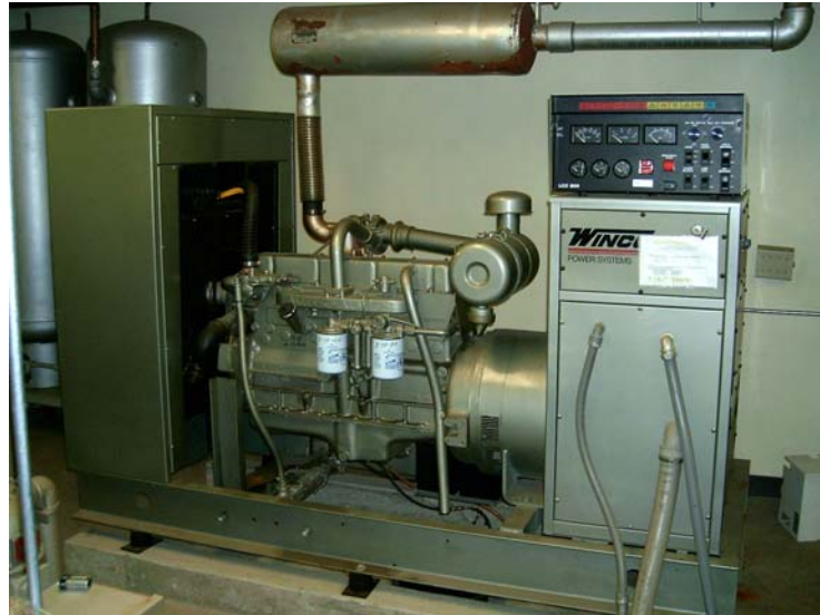
Photo 4-3 75kVA Diesel Engine Standby Generator
