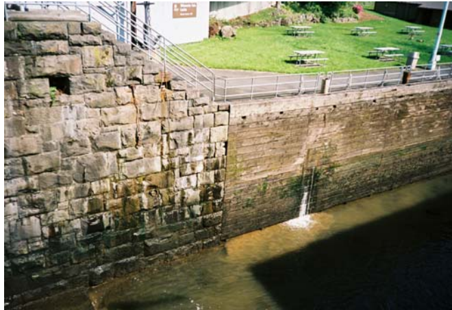
Photo 3-6 Through Wall Leakage (Landside) (Flow path extends beyond masonry)
