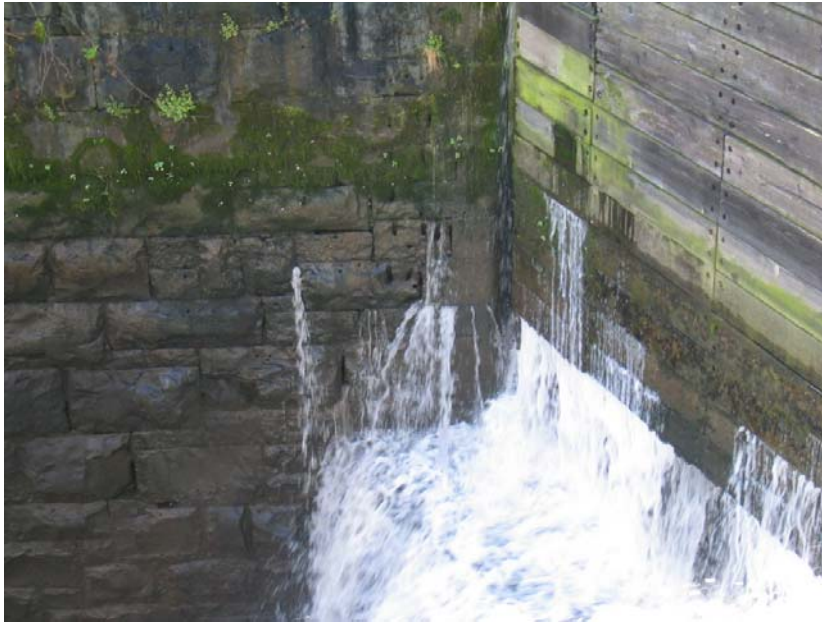
Photo 3-2 Through Wall Leakage (Riverside) (Flow rate increases and flow path lengthens as the chamber fills)
