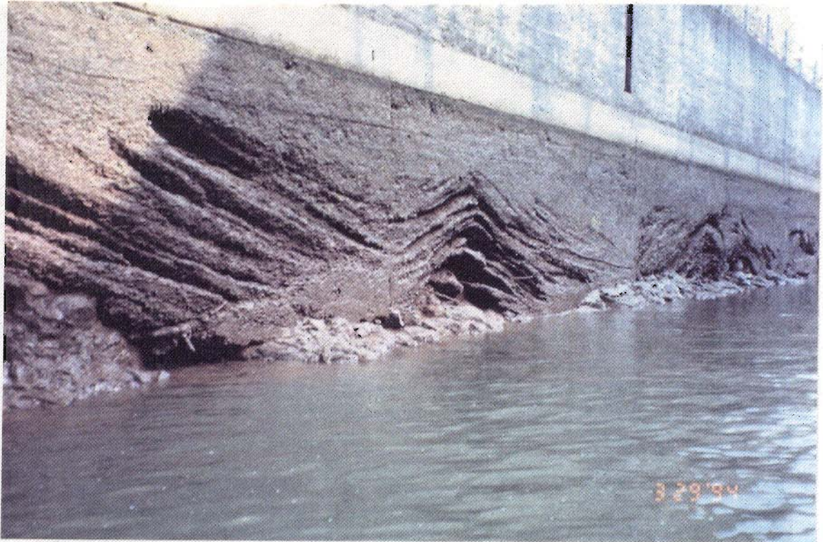
36. Left wall of guard lock, lower part of wall (ripples).
