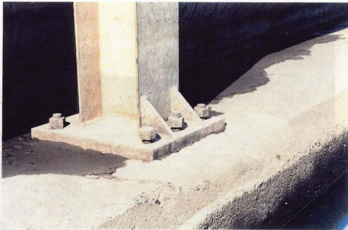
39. Downstream floating dock, upstream base on river side, loose nuts on anchor bolts.
