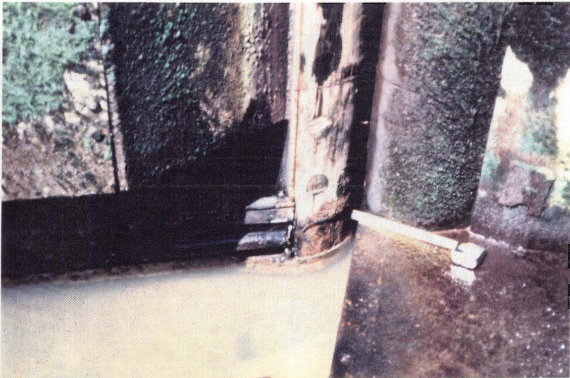
5. Gate 2, left side, gouge in quoin post (end of tape).
