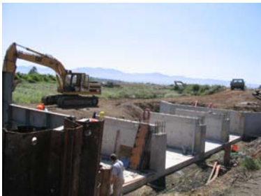
Construction of a new spillway in Tillamook
