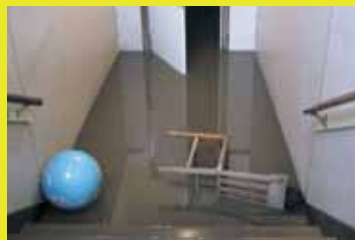
2007 floodwaters inundated the basement of Washington Grade School.
