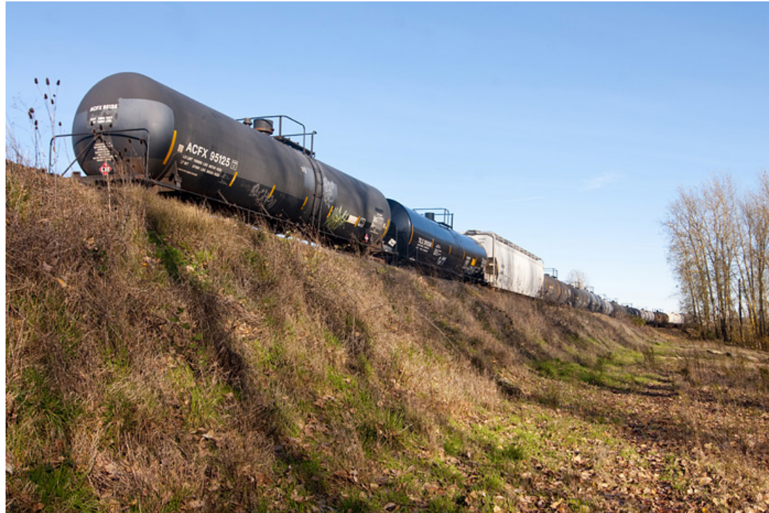
A railroad embankment near North Portland Road was the location of the breach that caused the Vanport flood in 1948. Parts of the berm have been identified by Levee Ready Columbia as needing improvement. (Sam Tenney/DJC)
