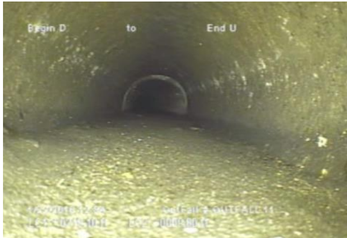
Outfall 11: settled deposits
