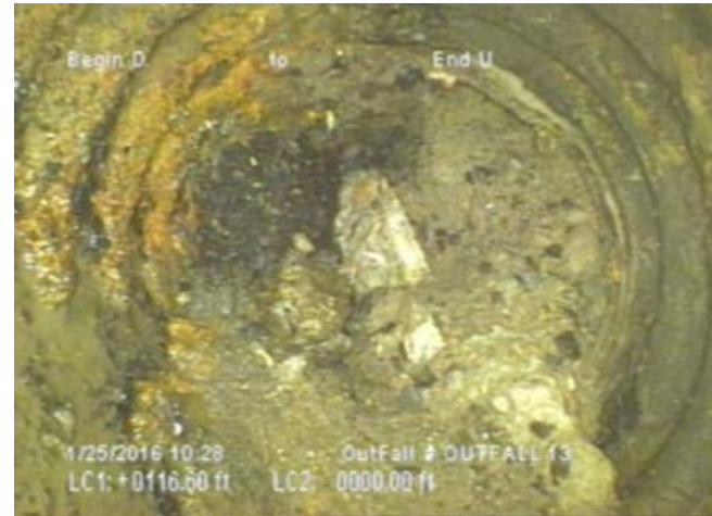
Outfall 13: heavy debris - 100% blockage
