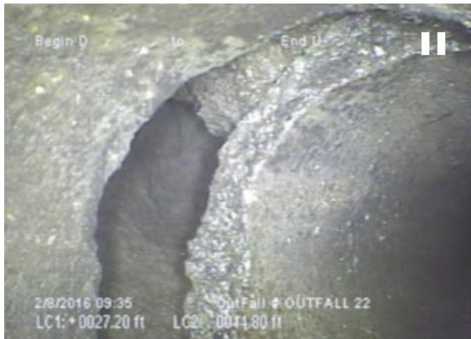
Outfall 22: open and offset joint
