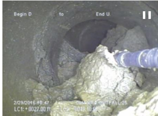
Outfall 25: broken pipe with heavy debris
