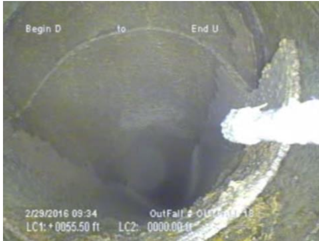
Outfall 18: broken pipe with steep grade break
