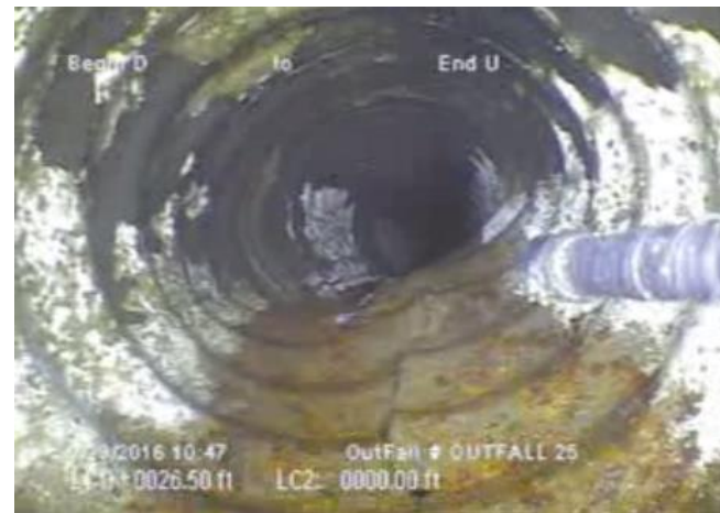
Outfall 25: deformed pipe
