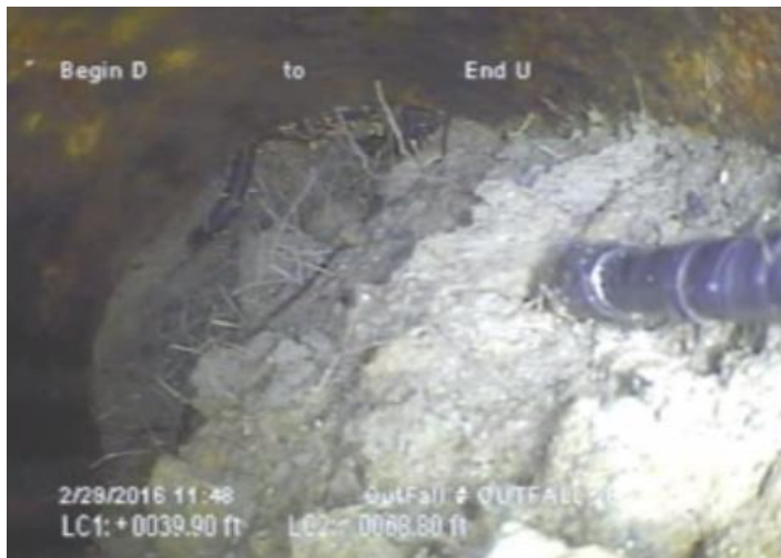
Outfall 28: heavy debris - 100% blockage with fine roots
