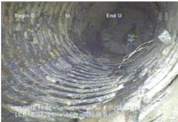
Outfall 29: surface reinforcement visible
