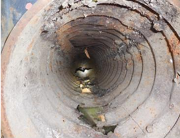
Outfall 10: holes with voids visible at discharge point
