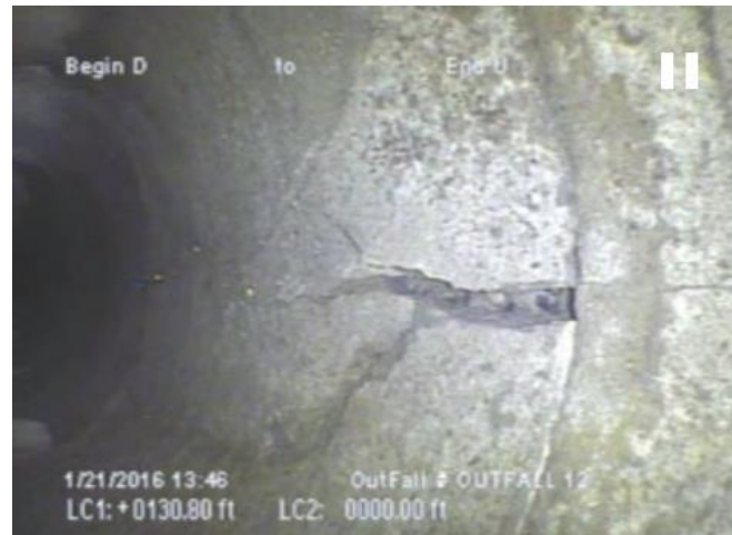
Outfall 12: broken pipe
