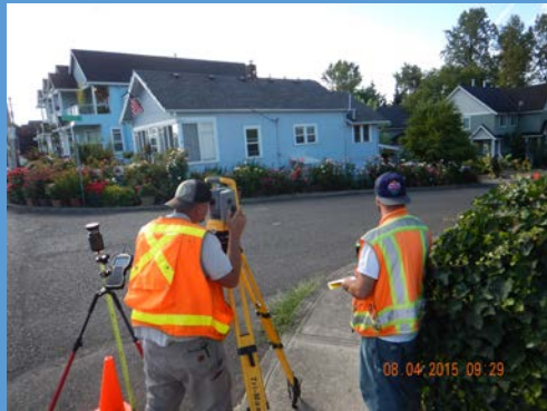
Surveyors capturing ground elevations along Bridgeton Road levee
