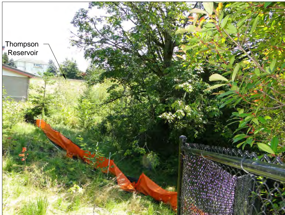
Photo 4: Facing southeast toward the Thompson Reservoir and Pump Station.
