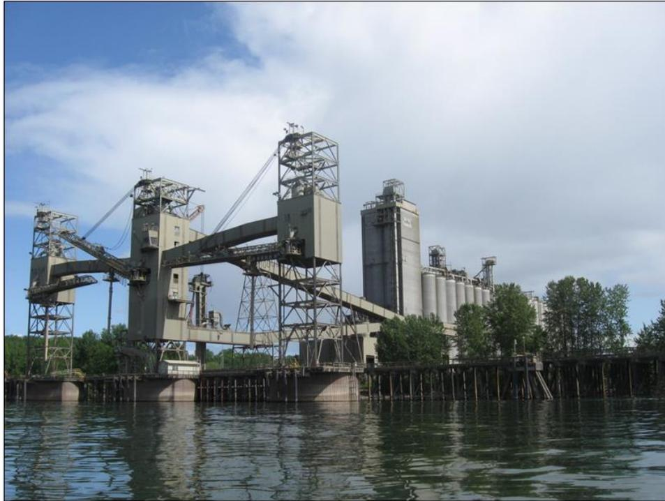
**Photo 3 – Berth 501 dock and shiploader towers general arrangement**
