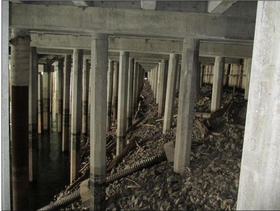
**Photo 2 – Berth 411 typical concrete piles and pile caps arrangement**
