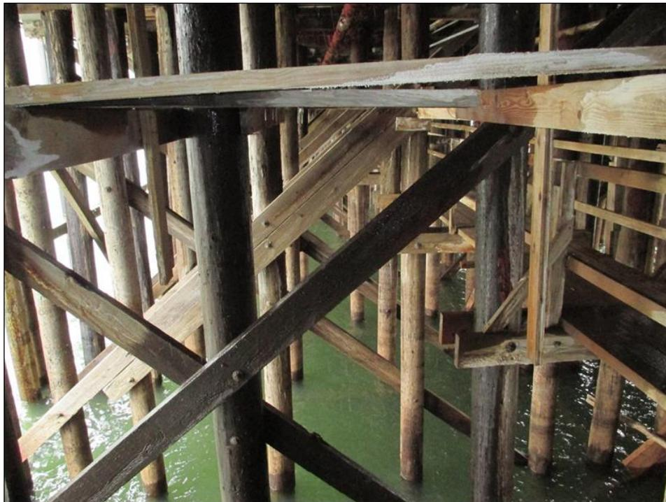
**Photo 1 – Berth 410 typical timber piles and bracing configuration**
