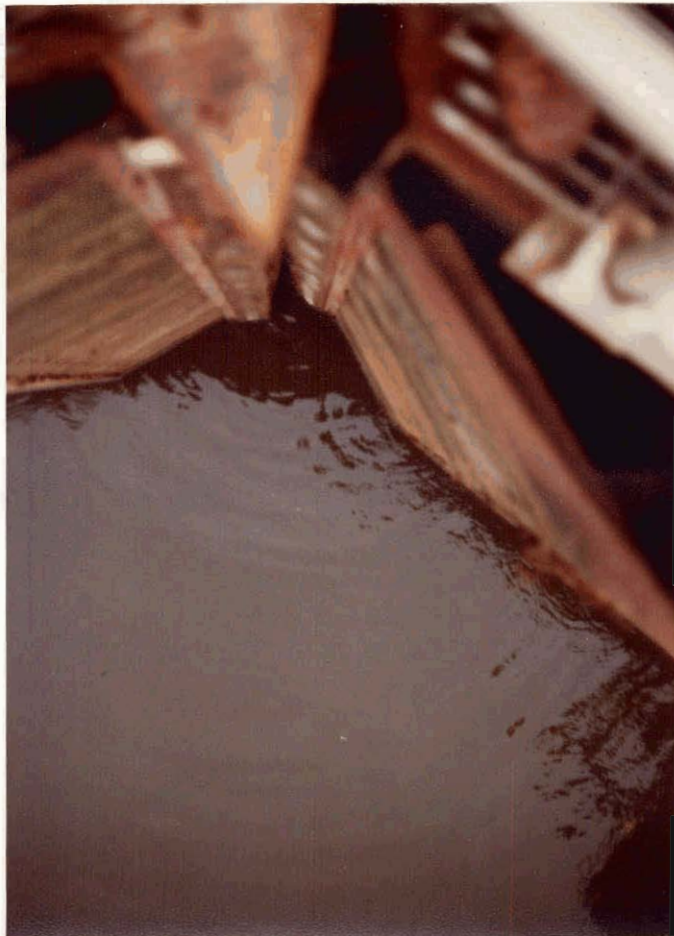
11 Feb 82 Gate No. 1 Willamette Falls Lock
