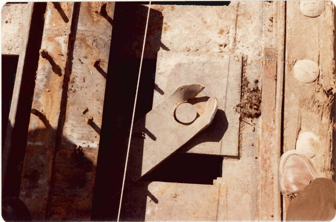
Frame (10) 5 May 82 Gate No. 1 Left Leaf - Lower end of Diagonal
