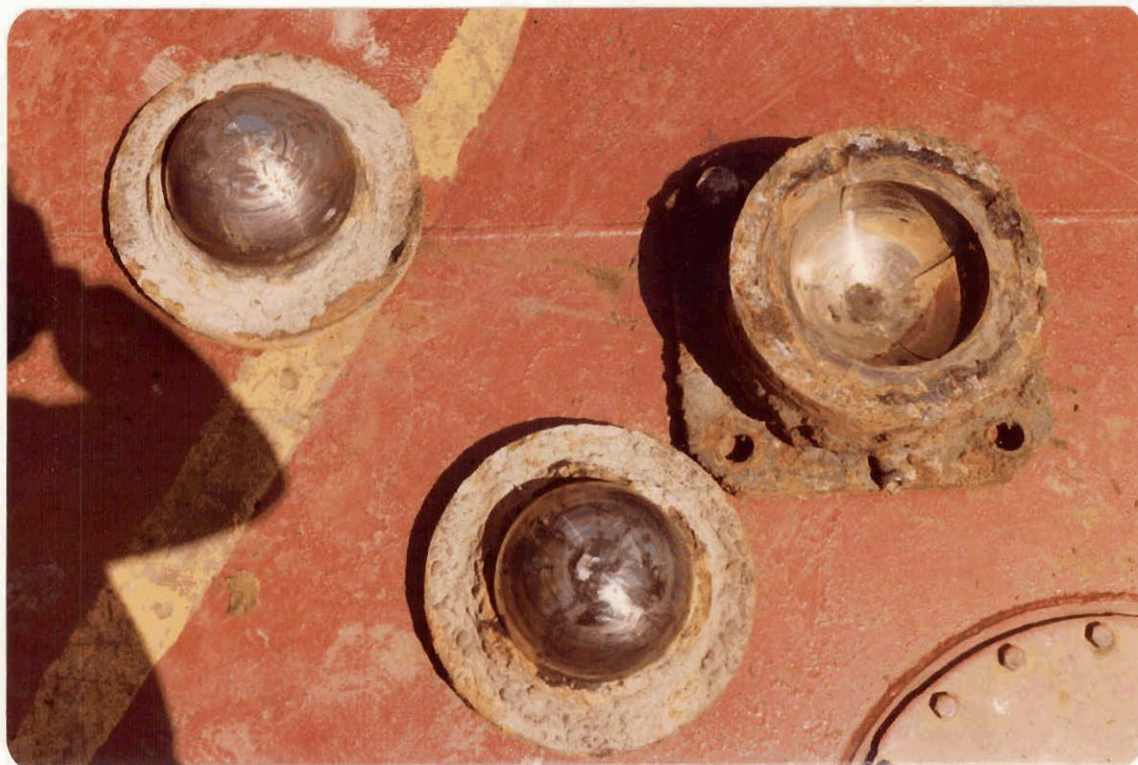
Frame ① 4 May 82 Gate No. 1 Pintles for Rt & Lt. Leaves Pintle Bushing for Lt. Leaf
