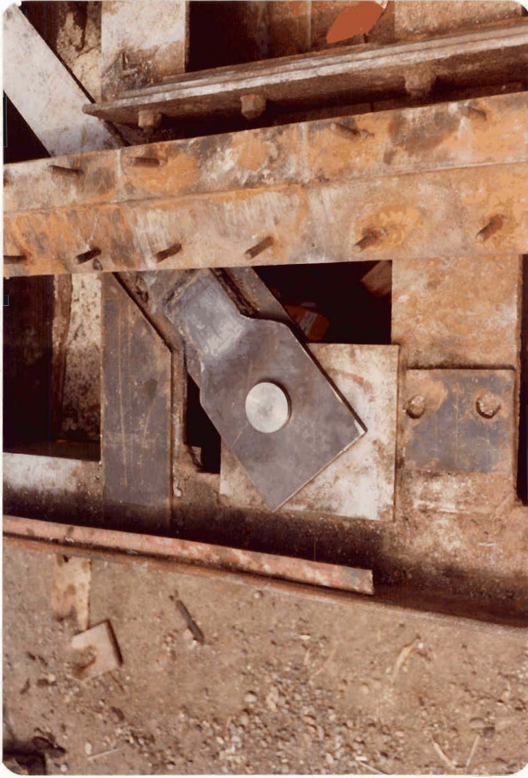
Frame 0A - Left Leaf - new diagonal eye at lower end. May 11, 1982
