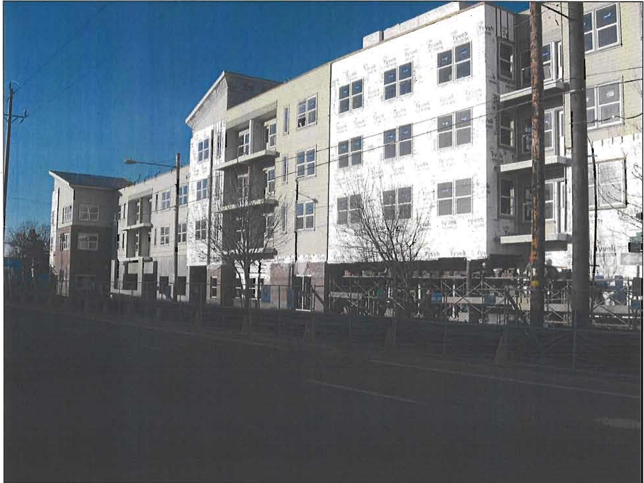
Figure 17. Humboldt Gardens under construction along Vancouver Avenue
