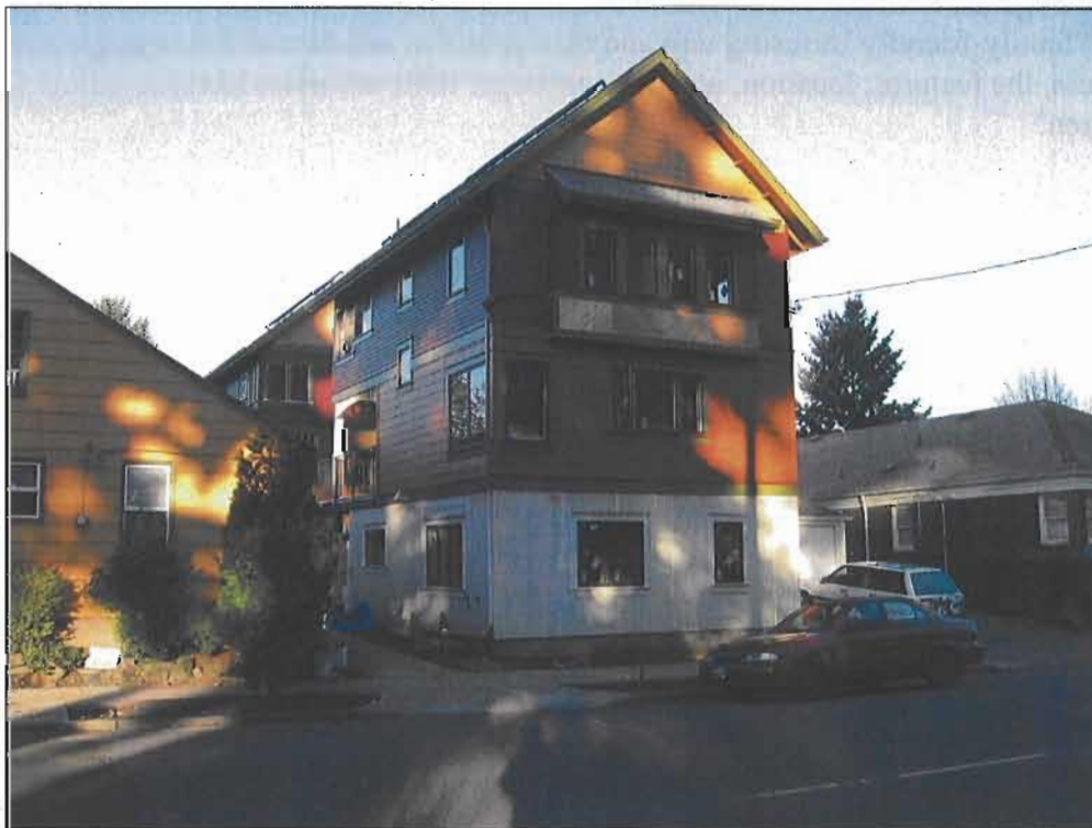
Figure 20. Peninsula Park Commons, North Lot, under construction.
